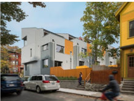
Rear Facade from Marcella Street - Photo Credit: Sam Oberter
