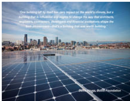
PV array - Photo Credit: Nic Lehoux
