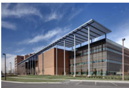
Canopy, brise soleil, and stepped footprint, south facade.
