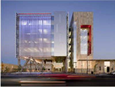
View of office tower from west - Photo Credit: SmithGroupJJR
