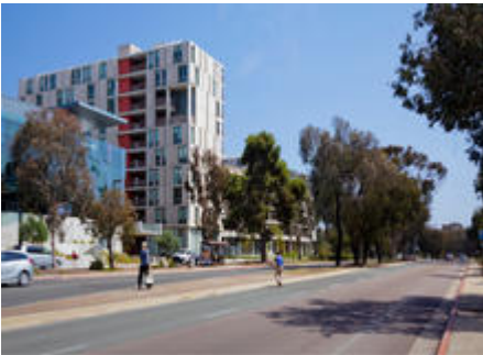
View looking south on Torrey Pines Road - Photo Credit: Tim Griffith
