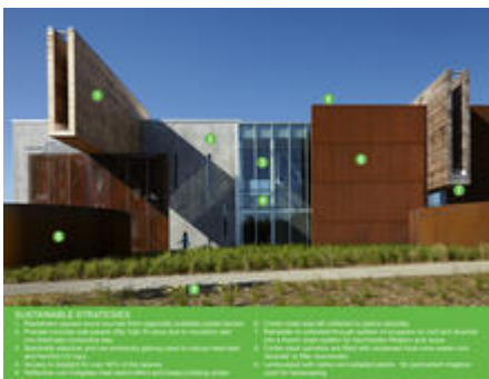
Exterior Sustainable Strategies - Photo Credit: Kate Joyce Studios with Legend by Ross Barney Architects
