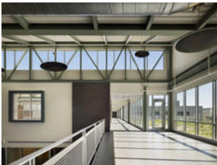
Daylighting with clerestories, skylights and borrowed light - Photo Credit: Barry Halkin, Halkin Photography
