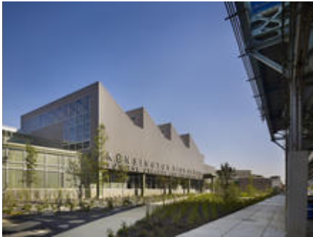
View looking south under EL - Fall 2010 - Photo Credit: Barry Halkin, Halkin Photography
