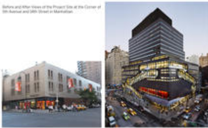
Before and After View of Project Site at 14th Street and 5th Avenue in Manhattan - Photo Credit: Photos © SOM (left) and James Ewing (right)
