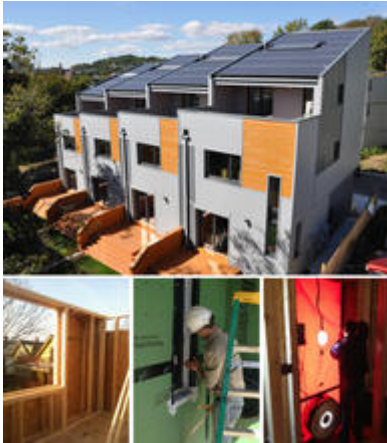
Clockwise from Top: View of Solar Array, Double Wall Construction, Air Sealing and Double Wall Construction - Photo Credit: Transformation Solar and Urbanica
