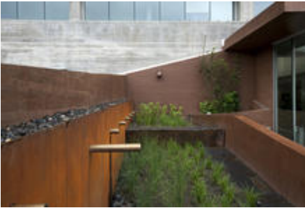
View of custom rainwater collection and stormwater treatment system. - Photo Credit: Sally Schoolmaster
