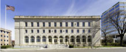
Wayne N. Aspinall Federal Building and U.S. Courthouse (South Elevation) - Photo Credit: Kevin G. Reeves, Photographer
