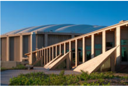
Green Roof - Photo Credit: David Lamb Photography
