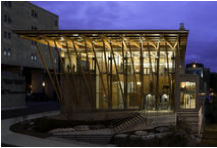
Main Entrance - Photo Credit: David Lamb Photography
