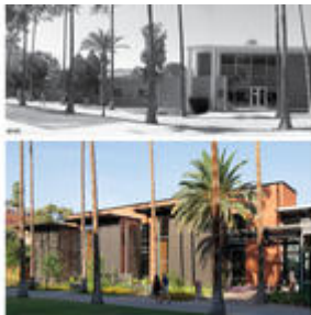
Adaptive reuse of the existing Health Services Building - Photo Credit: Bill Timmerman
