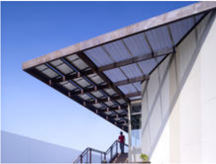
Detail of the large southwestern overhang with the 12kw solar system - Photo Credit: John Edward Linden
