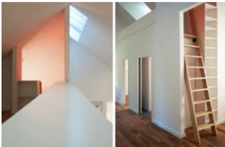
View from loft over top of marriage wall (left). Integrated ladder allows access to loft (right). - Photo Credit: Ken McCown
