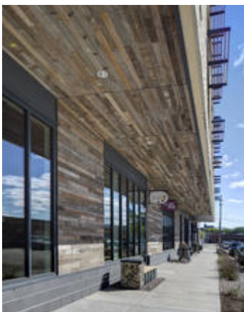
Overhang at South Facade -
